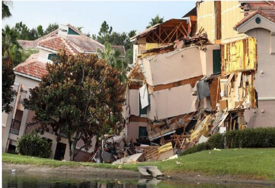
Buildings collapse into a sinkhole at the Summer Bay Resort on U.S. Highway 192 in Clermont, Florida. Guests had only 10 to 15 minutes to escape. The resort is located about 7 miles east of Walt Disney World. Red Huber/Orlando Sentinel/MCT
